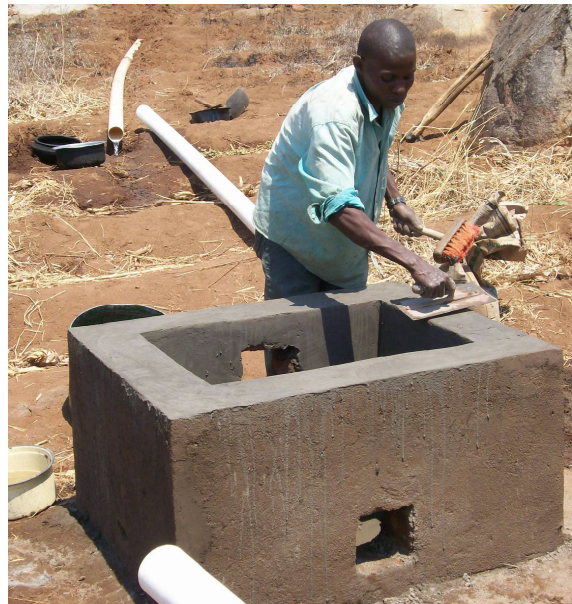
Constructing the irrigation scheme in Phalombe
